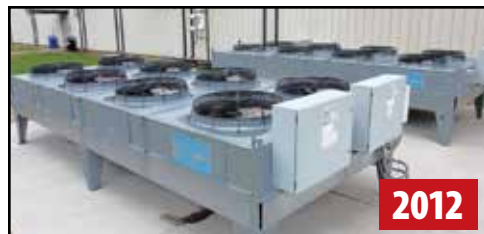
(2) THERMAL CARE LAVF-24410MA REMOTE CONDENSERS
