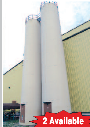
View of Silos
