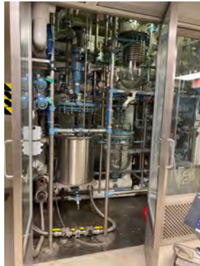
Multiple Kilo Lab Reactor Trains
